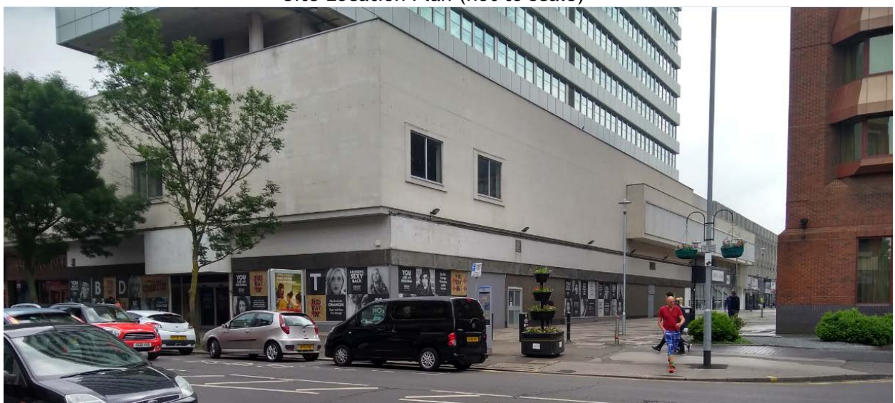
Site photograph showing the junction of Oxford Road and Queens Walk
